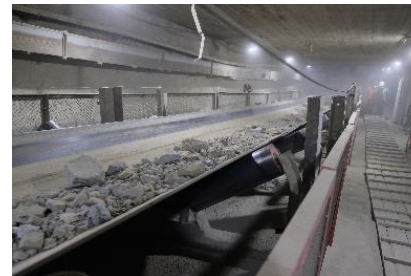
ORE CONVEYER SYSTEM AT DUKAT
